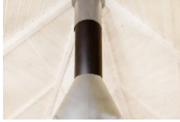
Grill Chimney Extension
