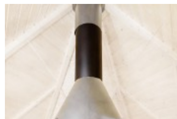
Grill Chimney Extension
